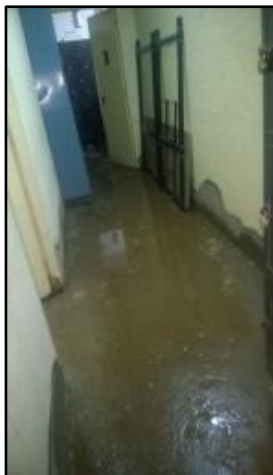
Fig 2 The basement passage started showing ground water dampness in 2010
