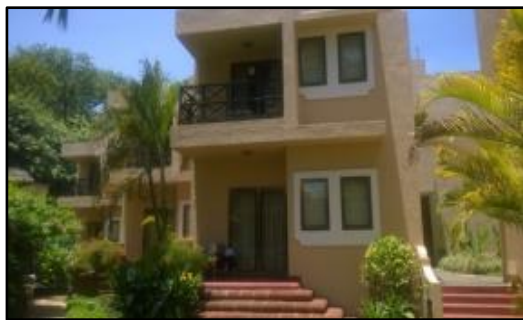
Fig 1 Photo showing the building at the resort & access to the basement
