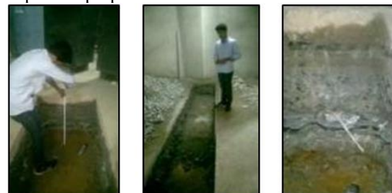
Fig 9 Inspection of open trench made in raft
