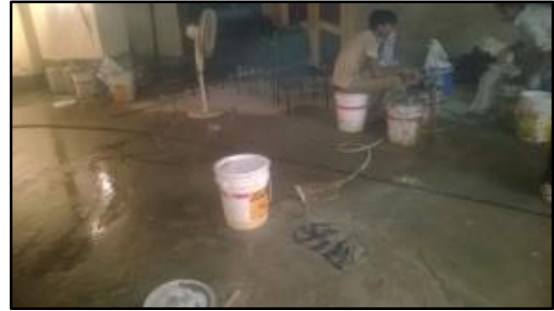
Fig 4 RCC raft treated with injection grout and waterproofing treatment in 2014.
