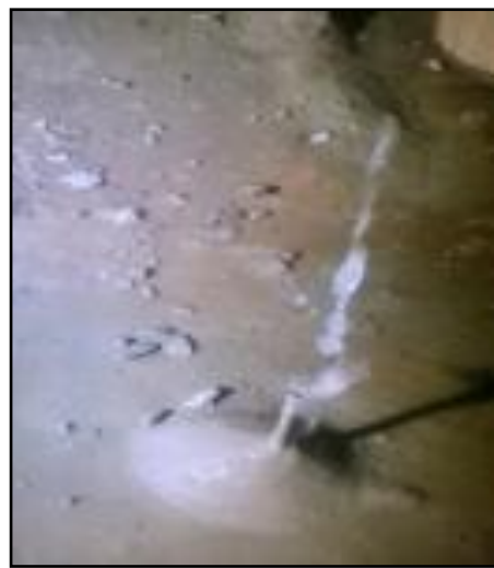
Fig 5 Underground water fountain out up to the height of 900 mm in Sept' 2015
