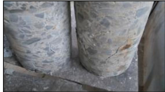
Fig 20 Failure of concrete core
